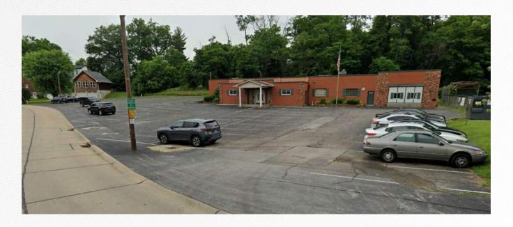
Asphalt pavement is in fair to poor condition and has slight to moderate cracks in 65-75% of overall surface.
